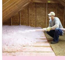
AttiCat<sup>®</sup> Expanding Blown-in Insulation Machine breaks up and conditions the AttiCat<sup>®</sup> Expanding Blown-in PINK<sup>®</sup> Fiberglas<sup>™</sup> Insulation throughout the length of the hose to increase insulating power.
